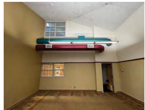
Paint existing walls and ductwork
