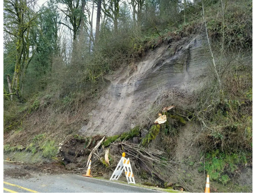
A landslide blocking East Pioneer Way in Puyallup, 2017.
