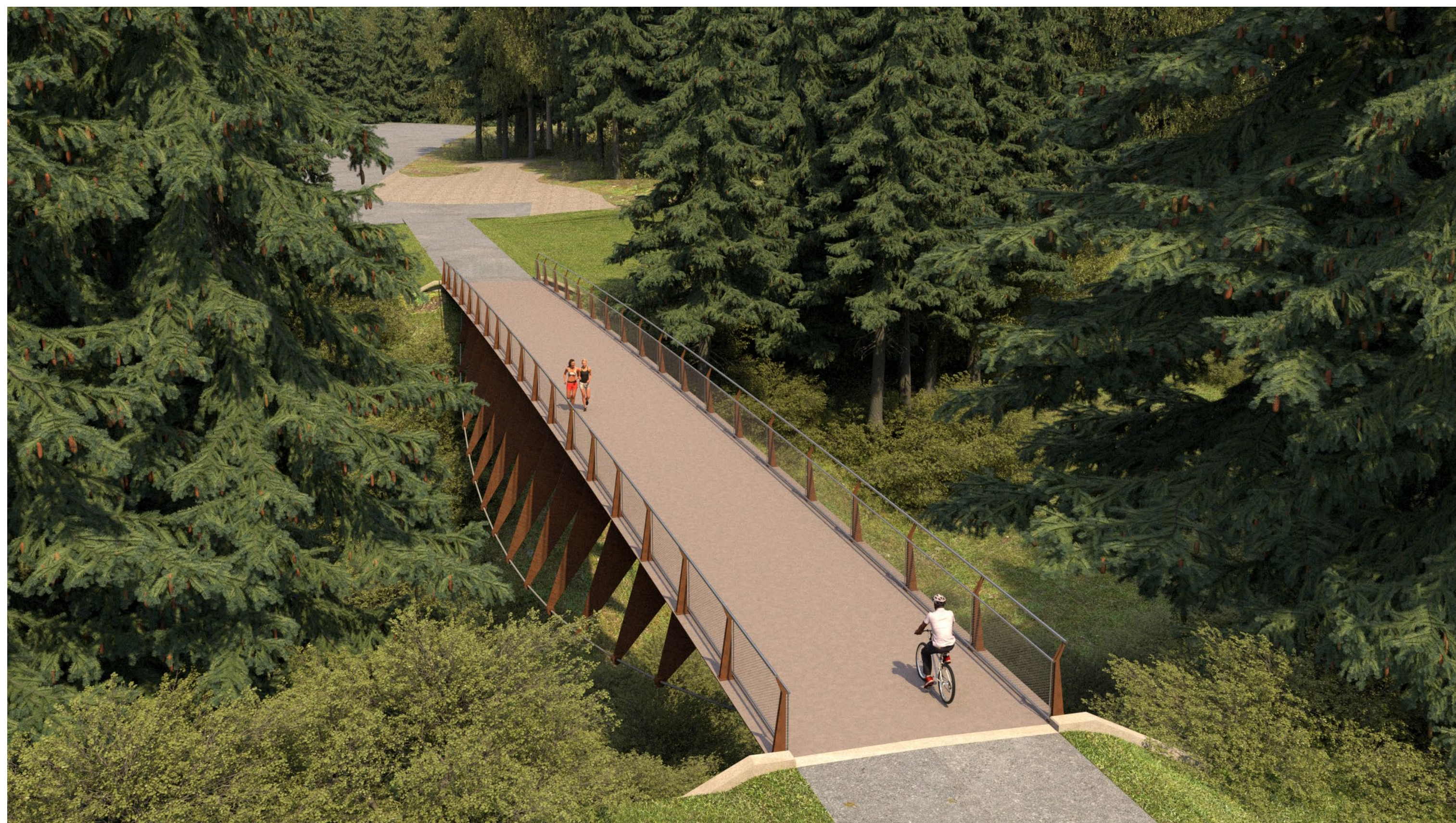
C - Underslung Bridge
