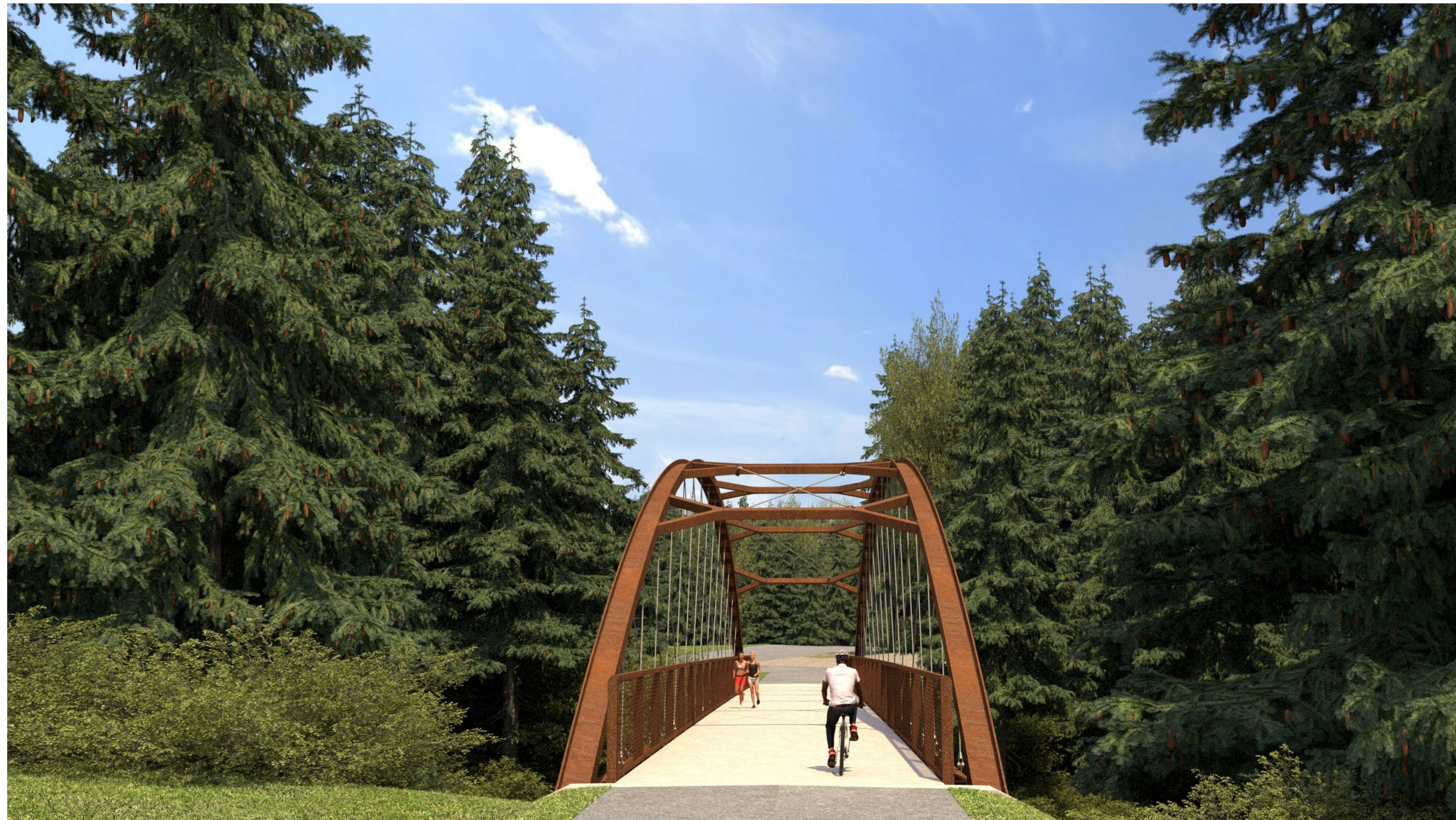
A - Arch Bridge
