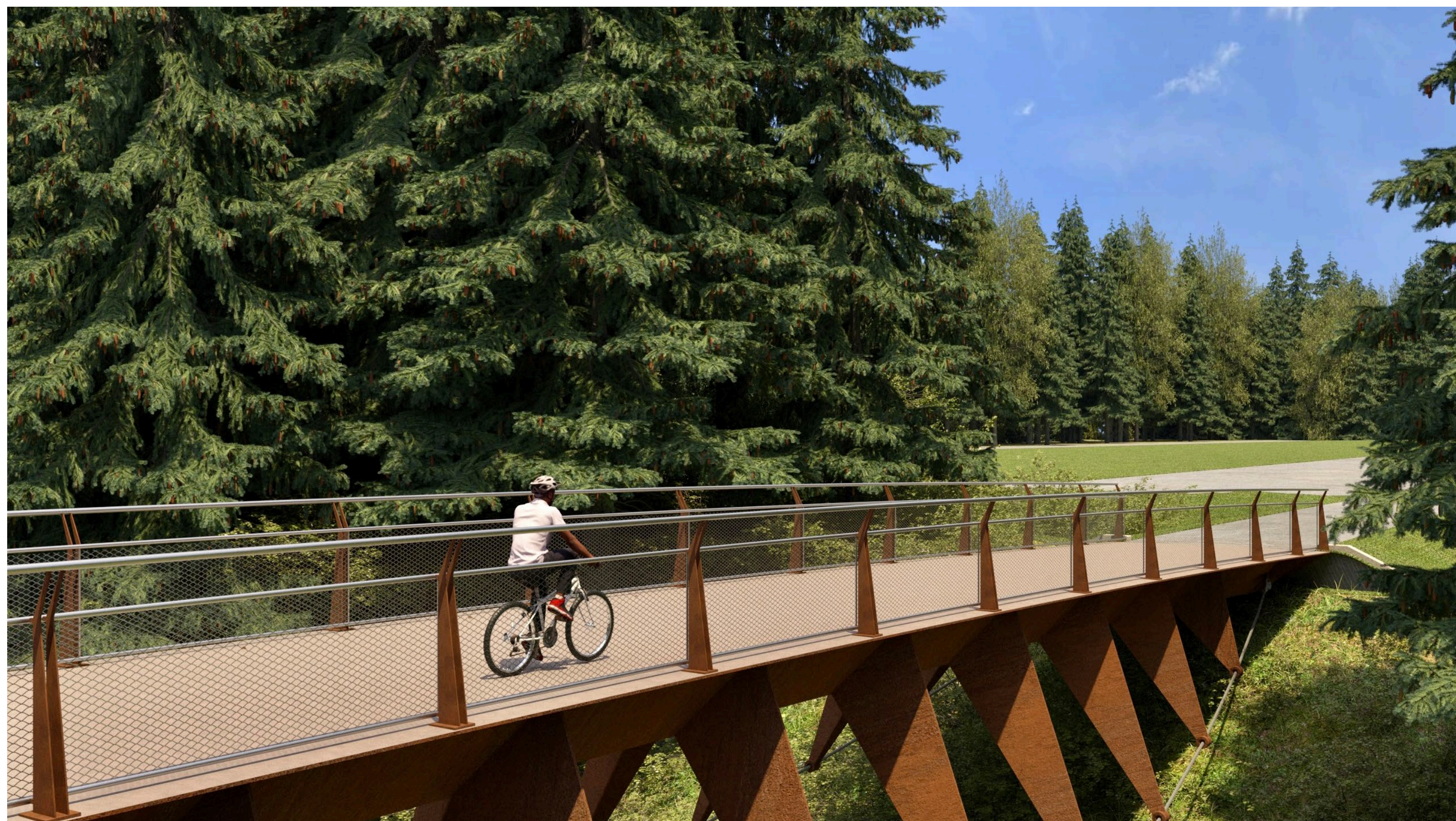
C - Underslung Bridge
