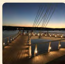
Integrated Walkway Lighting
